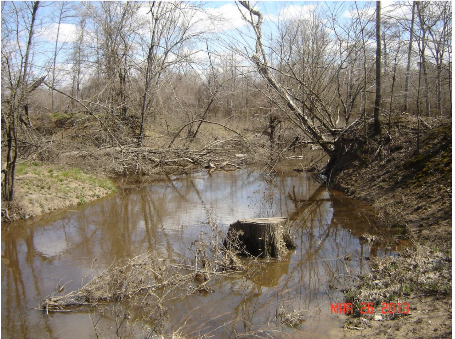
Timbered channel on west side of the site. Water was flowing from the Saline River through the channel on this date, 3-26/13.
